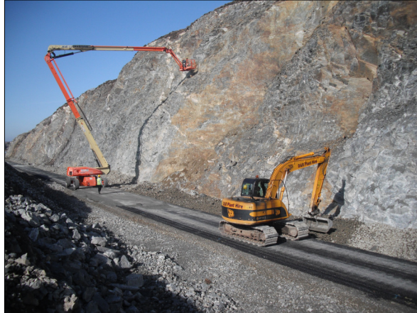
Work in Progress on N59 at Derrylea, Clifden
