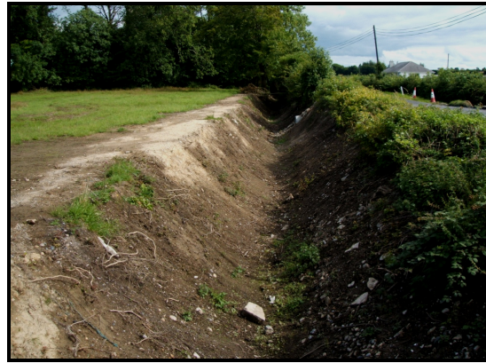
'After' – Remedial Works on Existing Drains
