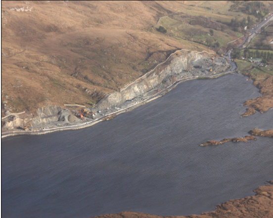
Aerial View of Work on N59 at Derrylea, Clifden
